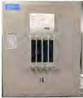
Photograph No. 34: 1S65 FL EV5 4.500 High Temperature
