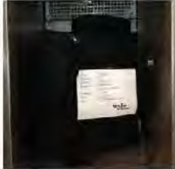
Photograph No. 33: 1S65 FL EV5 4.500 High Temperature
