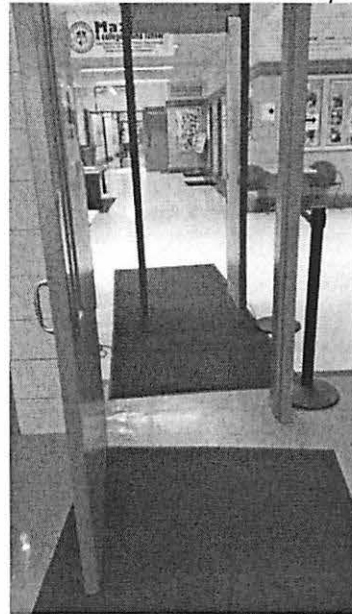
Photo #9. WH Maxwell – Security booth blocks access and narrows entryway.
