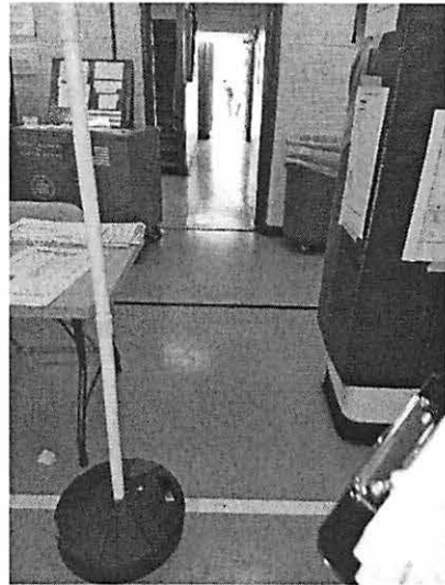
Photo #7. Authors Academy – Space too narrow to enter voting area with a wheelchair.
